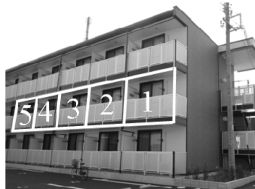
Fig. 2 Photograph of measured apartment.
